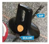
NOTE: When **FLASH**LOC is installed over gap between shingle tabs or vertical joints, fill gap/joint with sealant between mount and upslope edge of shingle course.
